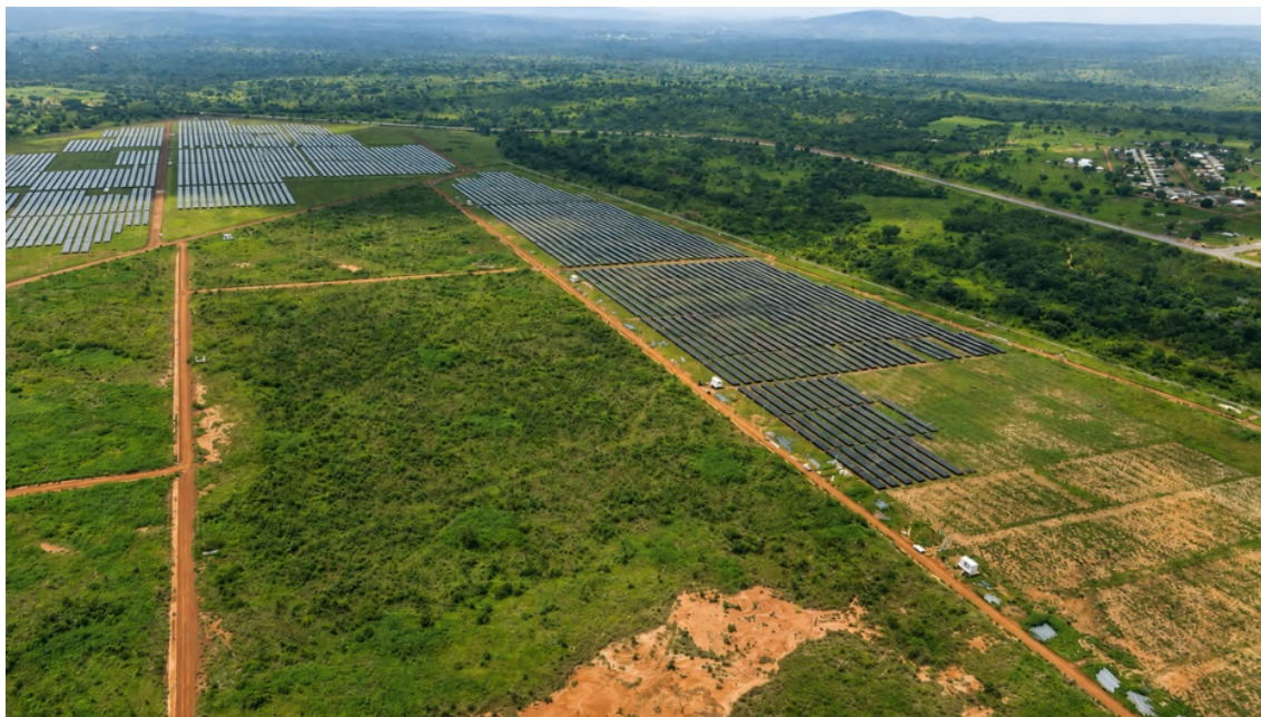
Figure 23 Aerial View of 100MWp Solar Plant at the Bui Generating Station
