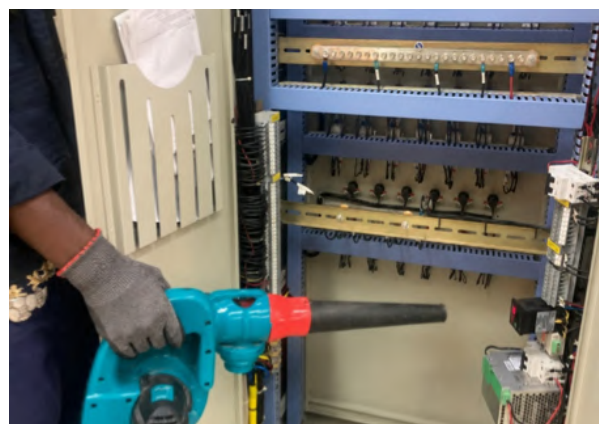
Figure 20 Blowing of Panels during Unit #1 Quarterly Maintenance Activities
