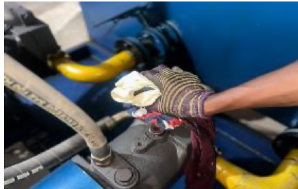
Figure 17 Cleaning and inspection of Unit 1 Intake gate hydraulic system
