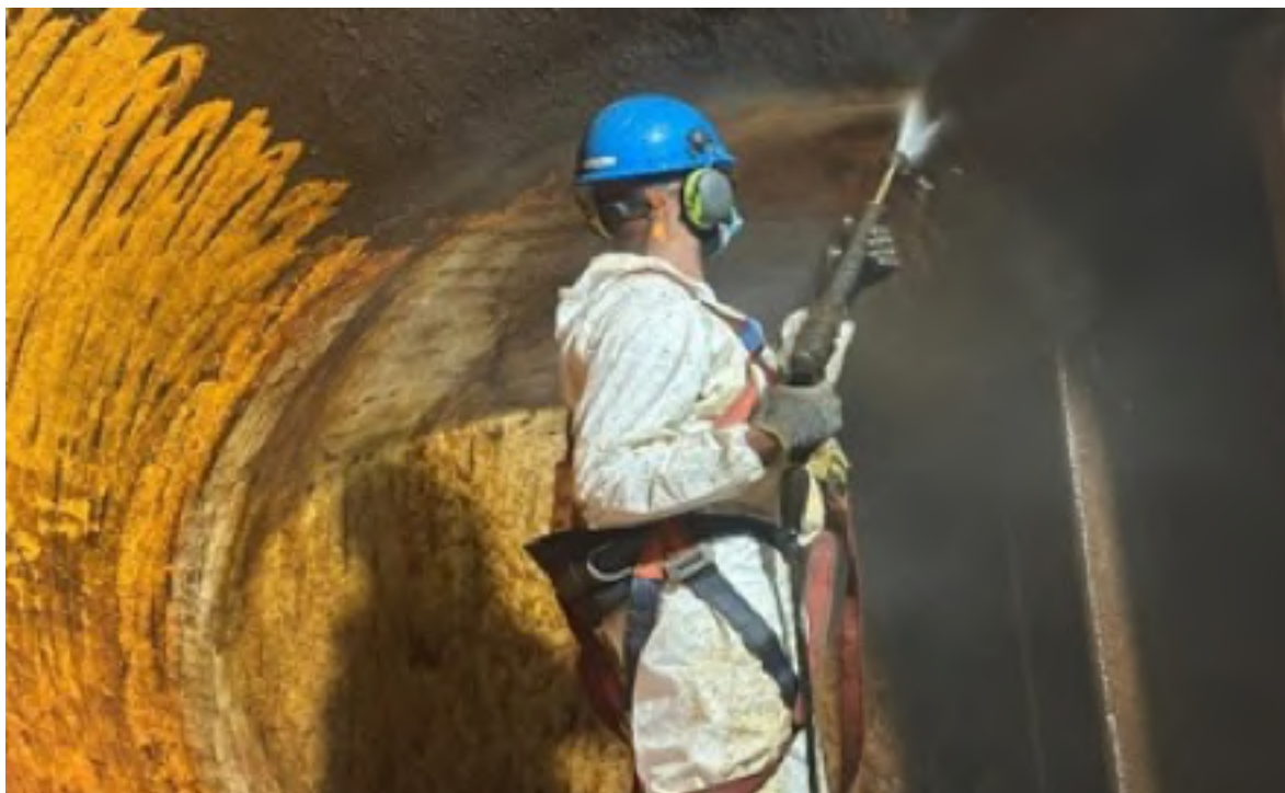
Figure 15 54G1- Cleaning of the interior of the Spiral Case
