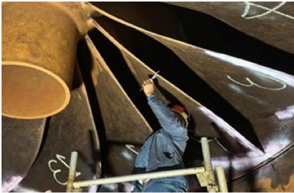
Figure 16 54G1- Wicket Gate Contact Clearance Checks
