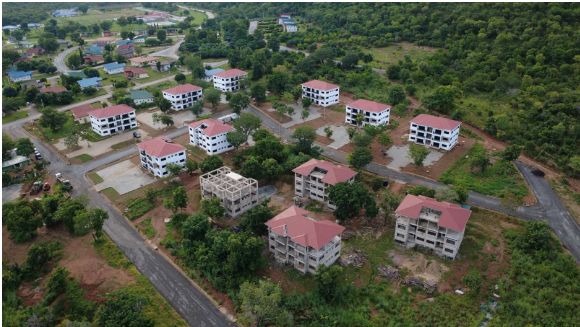
Figure 25 Aerial View of 2-Bedroom Staff Accommodation at the Village
