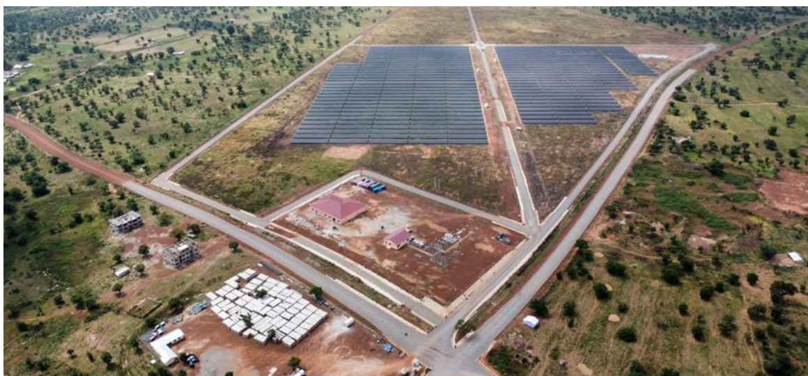
Figure 24 Aerial View of 50MWp Solar at Yendi
