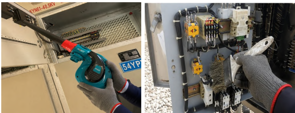
Figure 22 Blowing and Cleaning of accumulated dusts and dirt (Switchyard Monthly Maintenance)
